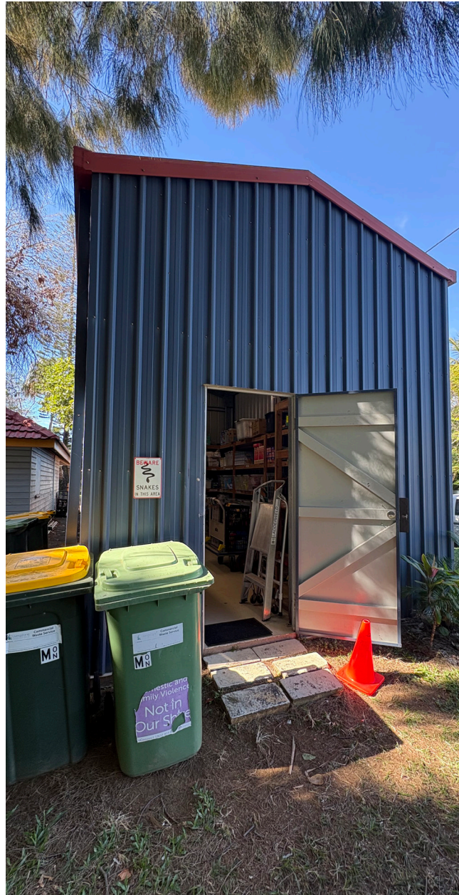
Exterior of the building / shed
